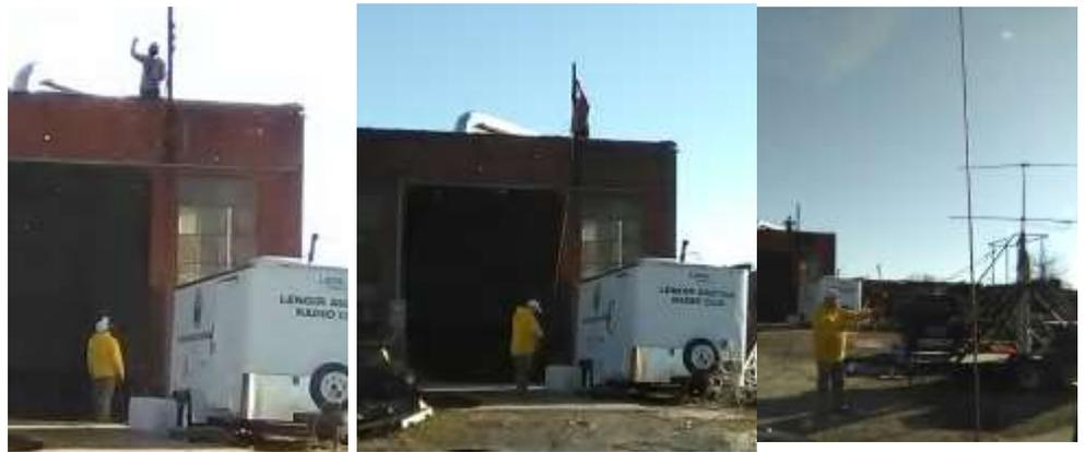
For this event, antennas for 2 meters, 6 meters, 20/40/80 were constructed. The radios that we were going to use were installed and tested. Propagation during the testing phase was great and gave us a glimpse into how things would go the next day.
