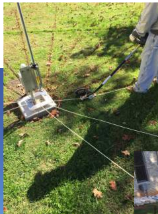
Vertical antenna mounted and radials buried.
